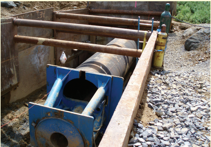
Tunnel being constructed under I-78 for conveyance of landfill gas to the generation station.
